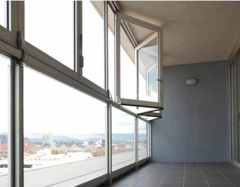
*Elevate™ Aluminium Systems Series 411 Bi-Fold with Centor E3 running gear adapted for Harkk Rect 86 Balustrade system*
